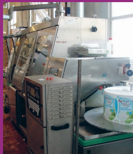
The EL1 filling line at Unimilk's Edelweis dairy in Kazan.
